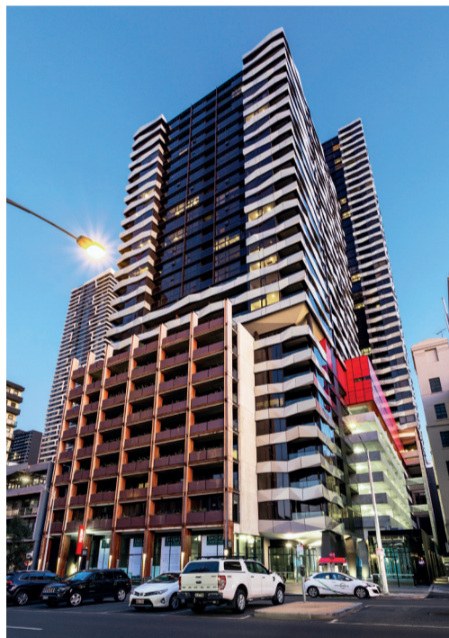
Right: The developer's first project in Australia, Fulton Lane on Franklin Street is a fully integrated mixed-use development situated in the heart of Melbourne CBD with 804 apartments in two residential towers and podiums atop a vibrant retail component
