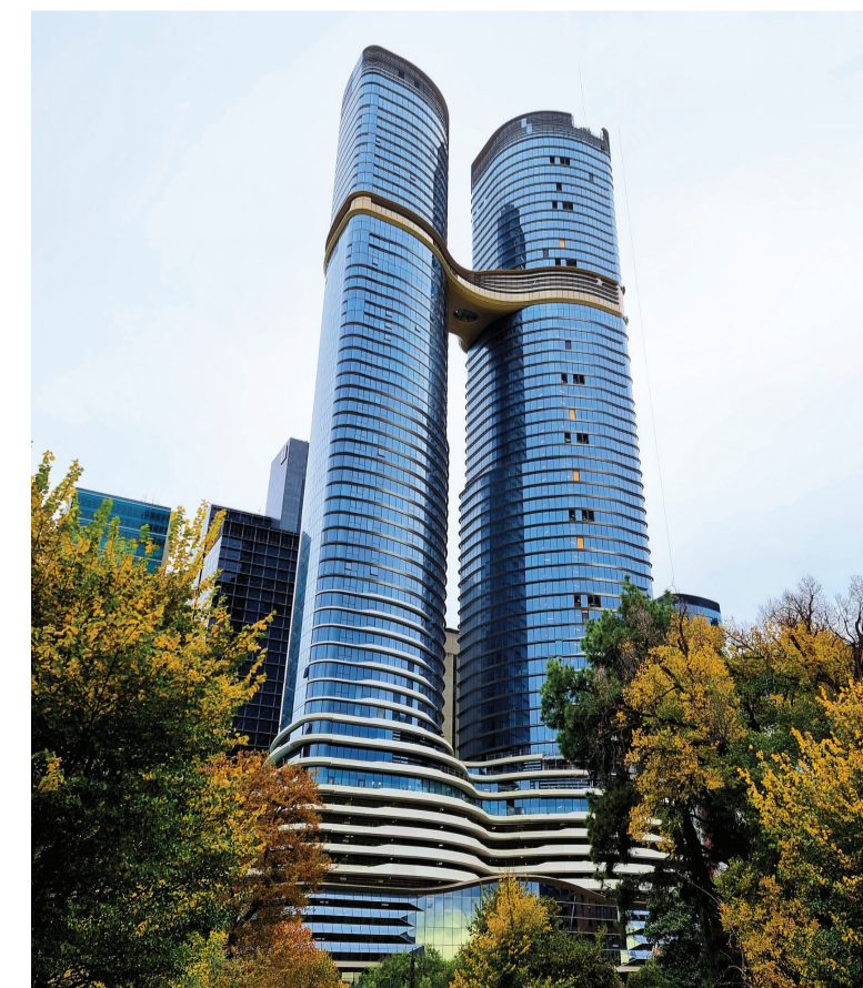
Sapphire by the Gardens on Exhibition Street will soon be home to Melbourne's first and much-anticipated Shangri-La Hotel. All 325 apartments in the residential tower are fully sold.
