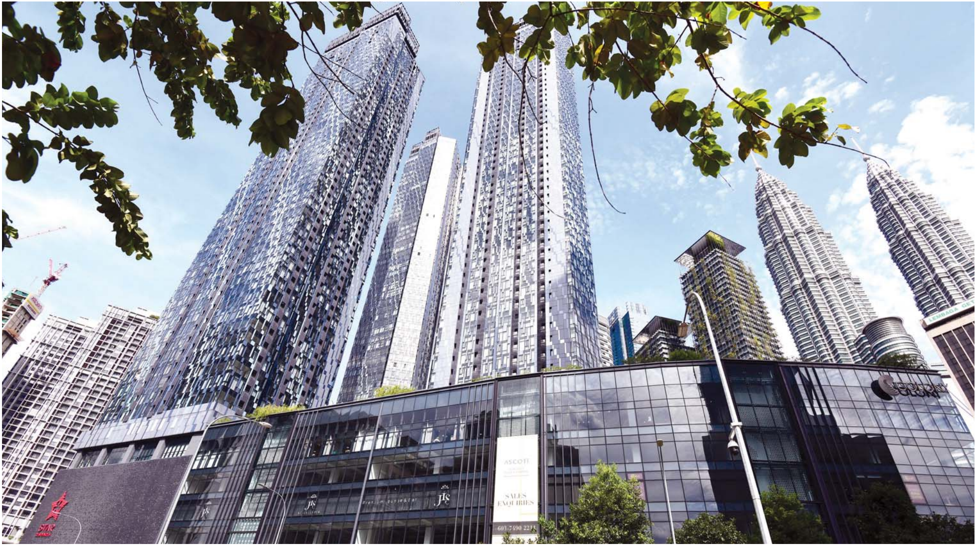
The podium façade is made from 88,000 pieces of 304 stainless steel plates
